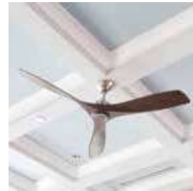
CEILING OIL BOUND DISTEMPER
