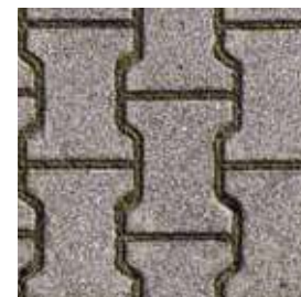
INTERNAL ROADS INTERLOCKING BLOCKS/ TREMIX CONCRETE ROAD
